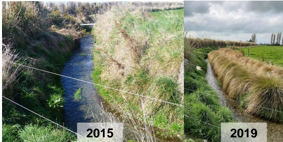
Figure 2: Waimanu Farm Stream Restoration Before and After Rebattering and Planting
